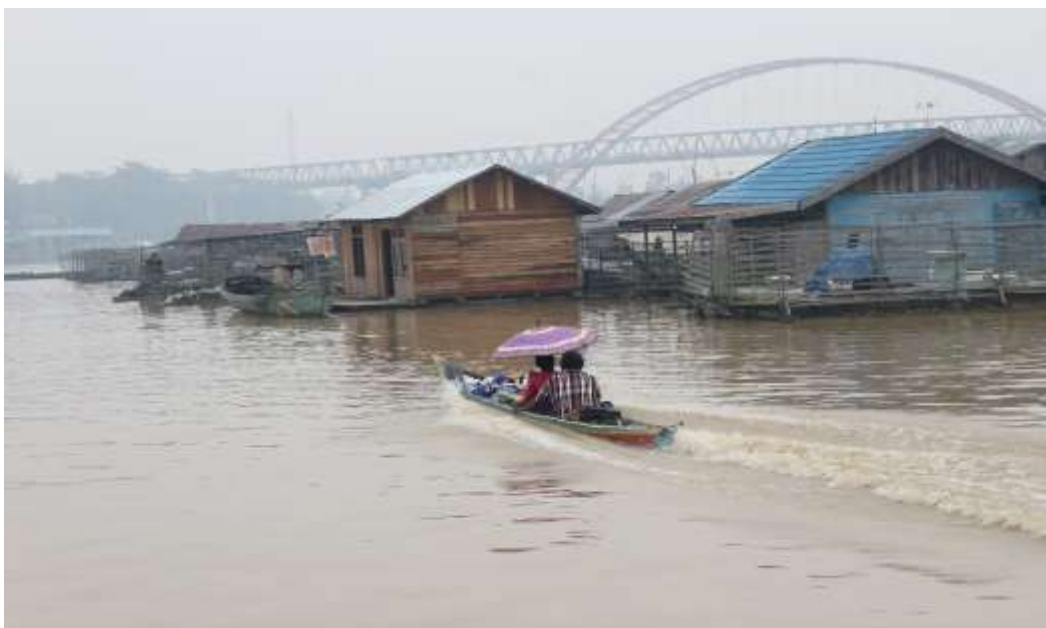
Figure 1 Kahayan Bridge Passing Over Kahayan River and A Row of Floating Houses
