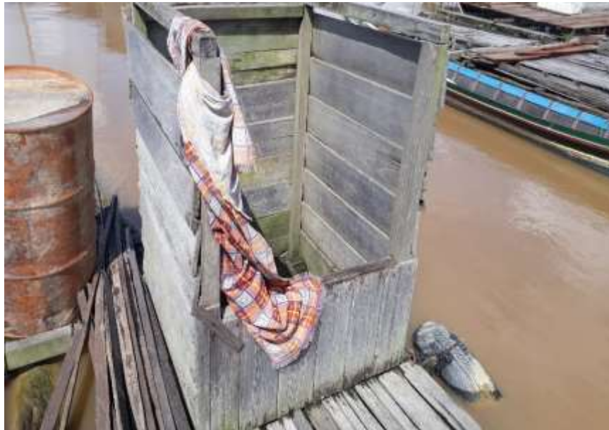
Figure 7 Floating Toilet on The River
